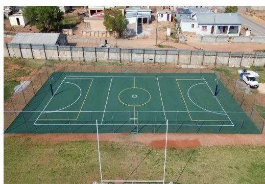
Photo: New Netball court construction Zolani, Ashton.
