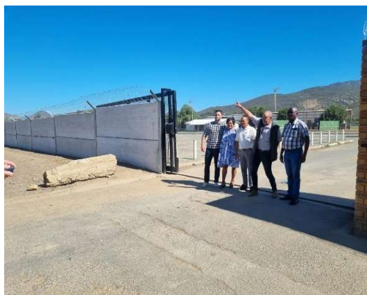
Photo: Van Zyl Street sport ground new precast boundary wall completed.
