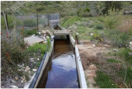
Raw water canal from Houtbaais River
