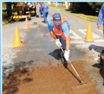
Ashbury road upgraded
