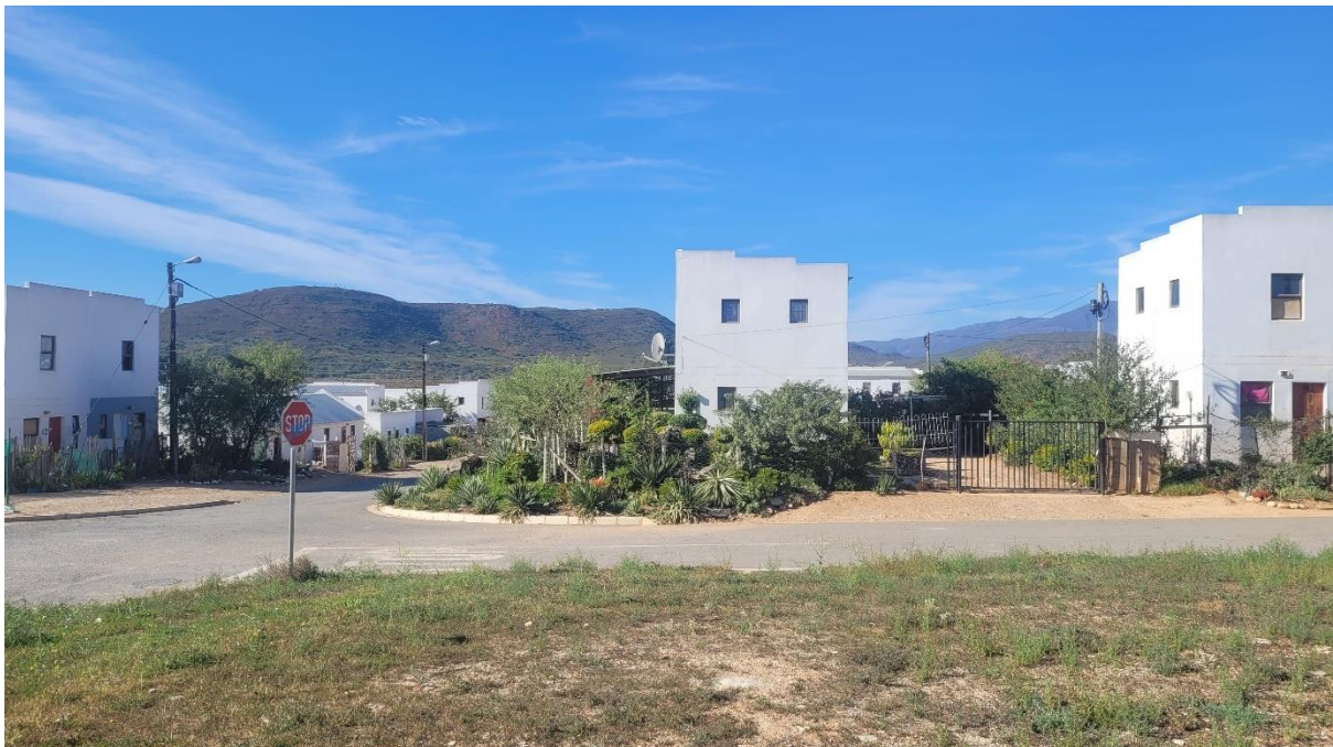
Figure 6.16: Front view of houses in White City
