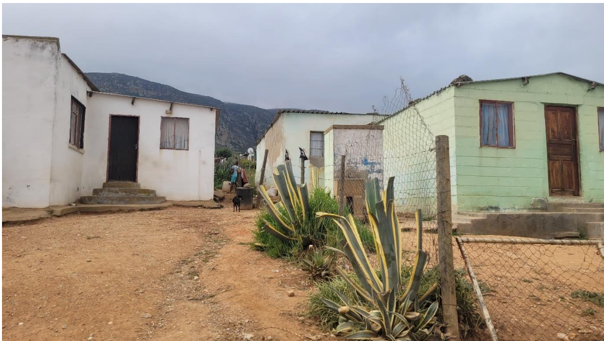
Figure 6.23: Houses in north-eastern Zolani
