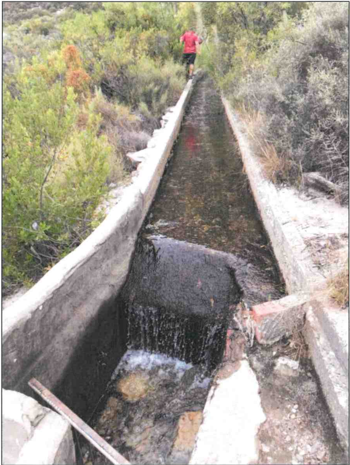
Portion of the old concrete water furrow
