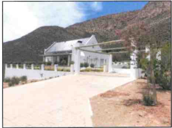
EXISTING MANAGER'S HOUSE
