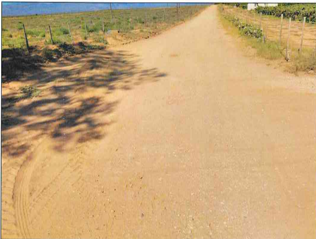
Figure 4: Public gravel road in very good condition
