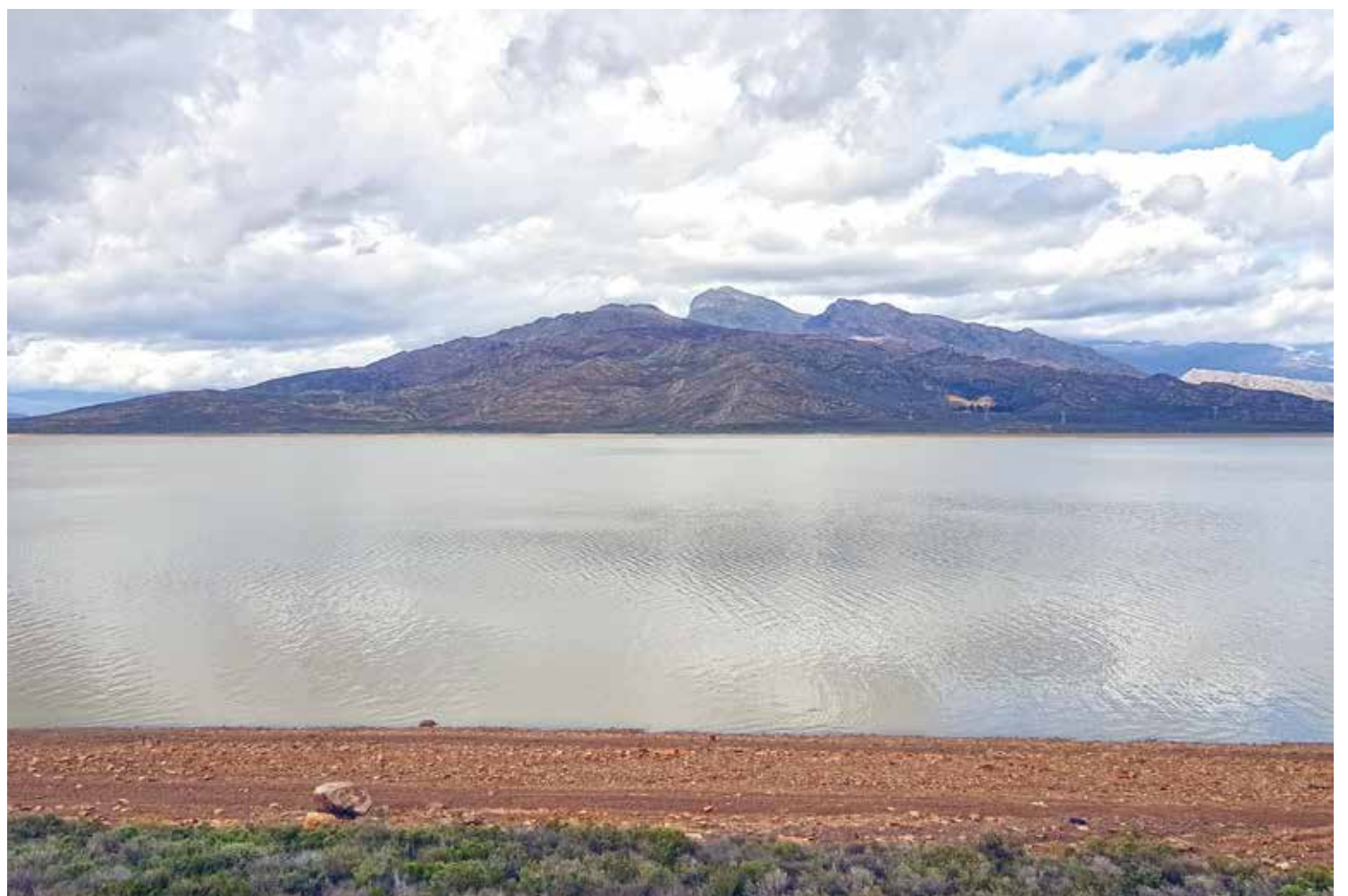
Low dam level: The Brandvlei dam level is under strain.
