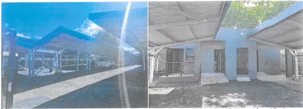
Upgrading of Robertson Informal Trading area
