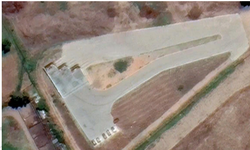
Robertson Transfer station
